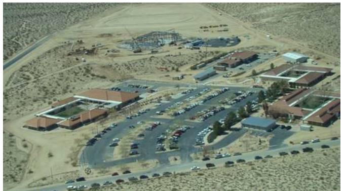
Campus Expansion: Start of Bell Center Construction, 2009
