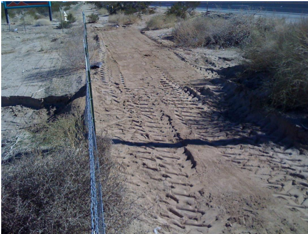
Photo Exhibit 2. Repair of TA fenceline, 21 January 2011.
