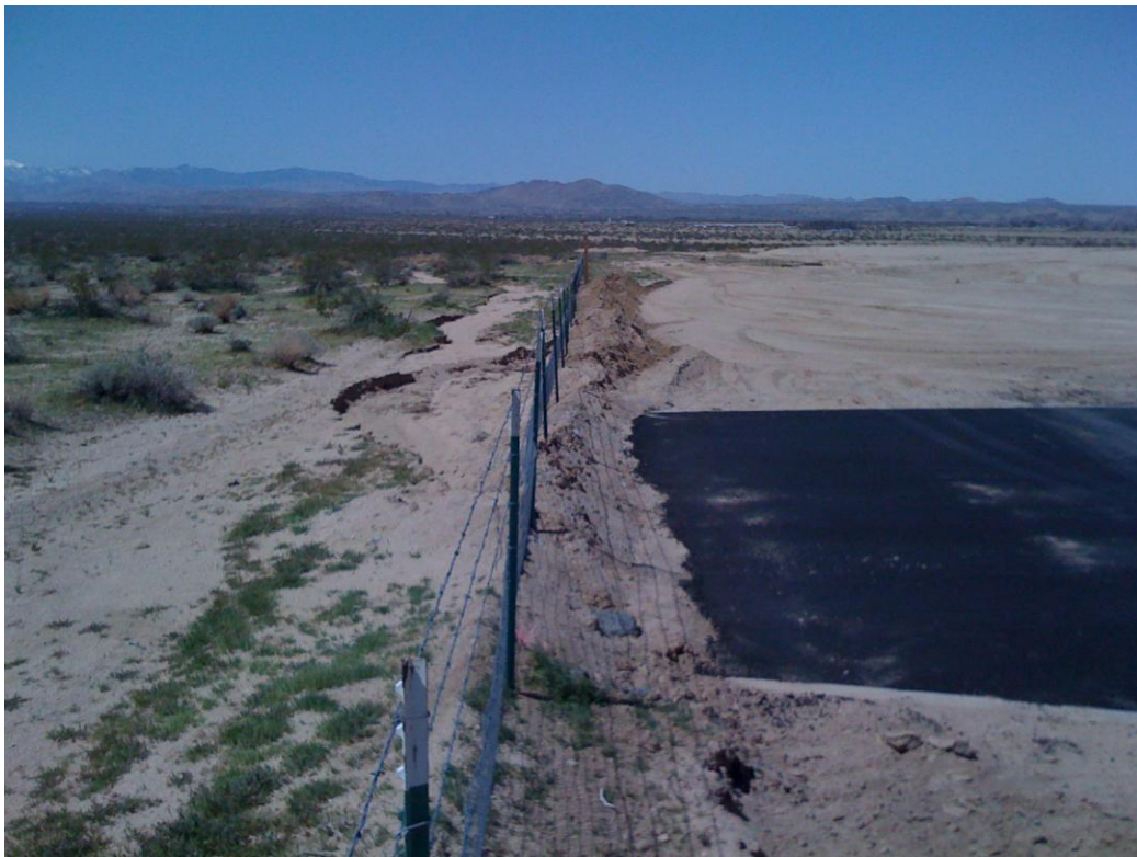
Photo Exhibit 2. Repaired fenceline of Translocation Area at Lewis Drive.
